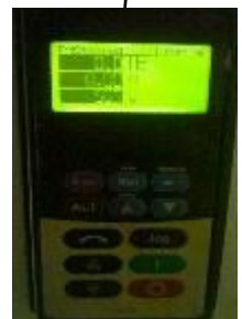
Pump Frequency adjustment at panel display
